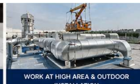
WORK AT HIGH AREA & OUTDOOR INSTALLATION
